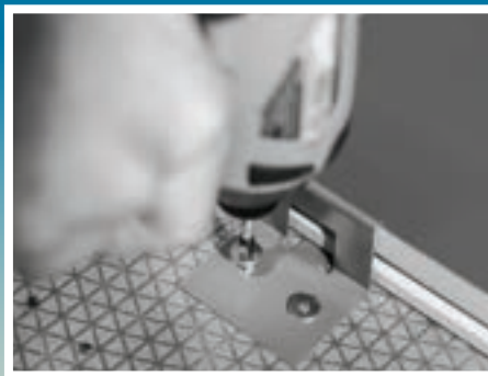
Fasten the hidden clip with pancake screws.
